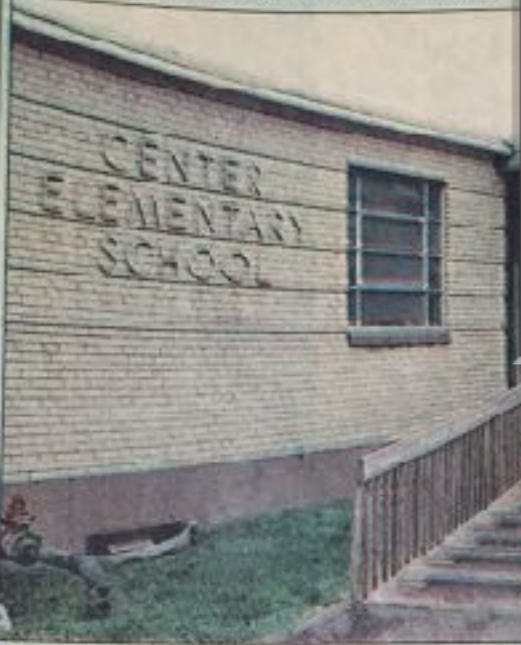
The renovation of Center Elementary School will cost between $7 million and $9 million. A new gym, library and six to 10 new classrooms are needed.
